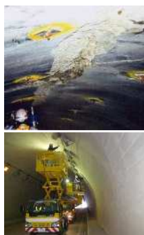
Inspection and diagnosis of tunnels
